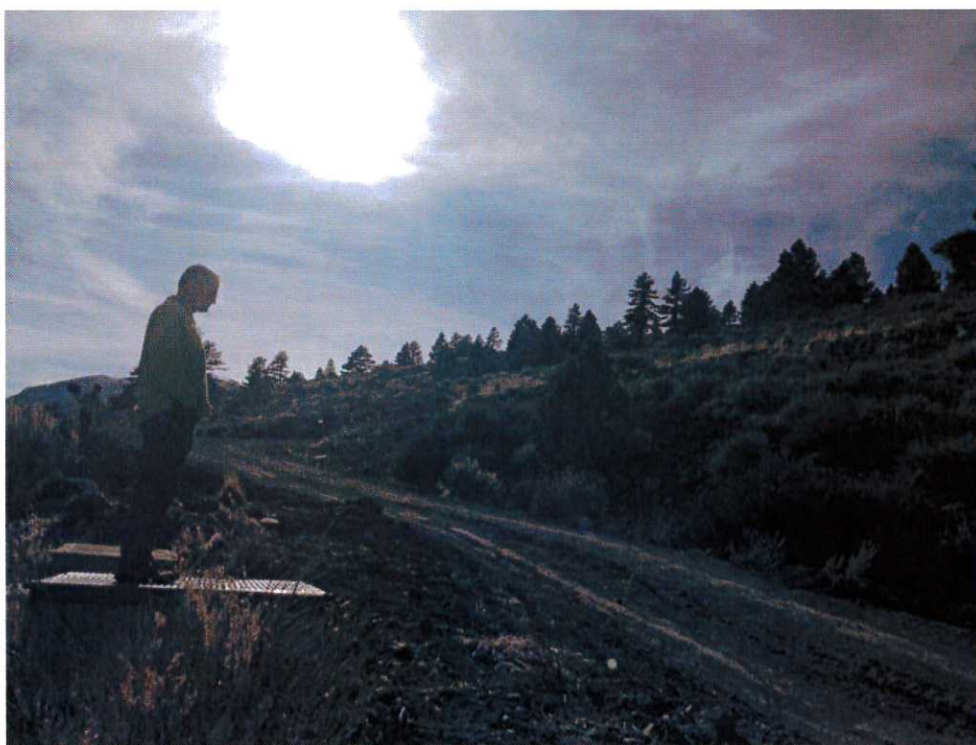
Power and Telco
